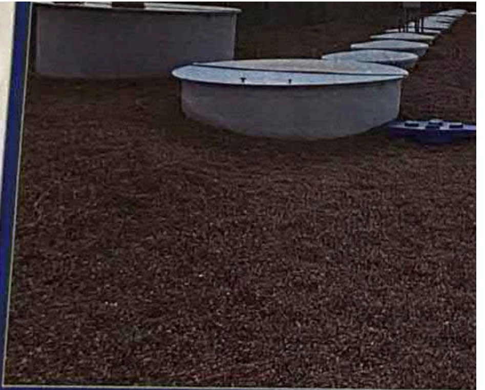
Wastewater Treatment P
